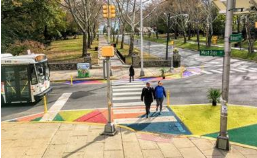
Example from City of Jersey of paint to expand pavement widths
